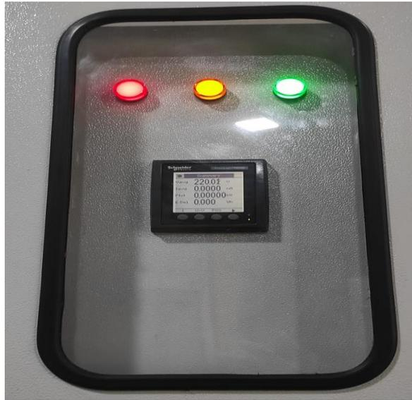
Gambar 8. Tampilan *Power Monitoring Panel AC COMBINER LVMDP*.
